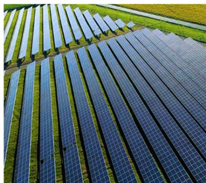
FREEMONT COMMUNITY SCHOOLS - SOLAR FARM
