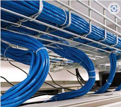
MCCORMICK & COMPANY - LEED V4.1
