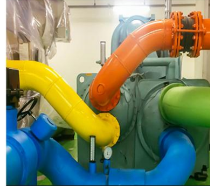
MOLINA HEALTHCARE - HVAC RETROFIT
