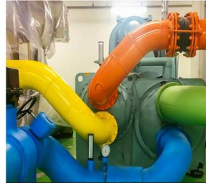
MOLINA HEALTHCARE - HVAC RETROFIT
